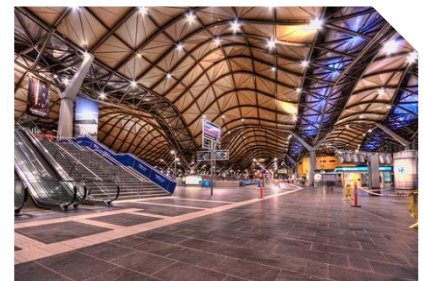
Southern Cross Station (Honeywell)
